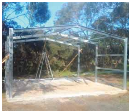
Shed framed up ready for sheeting
